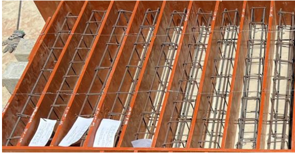
Fig. 8. Formwork and reinforcement processing
