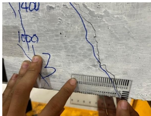
Fig. 31. Measure the crack width of D8 reinforced concrete beam
